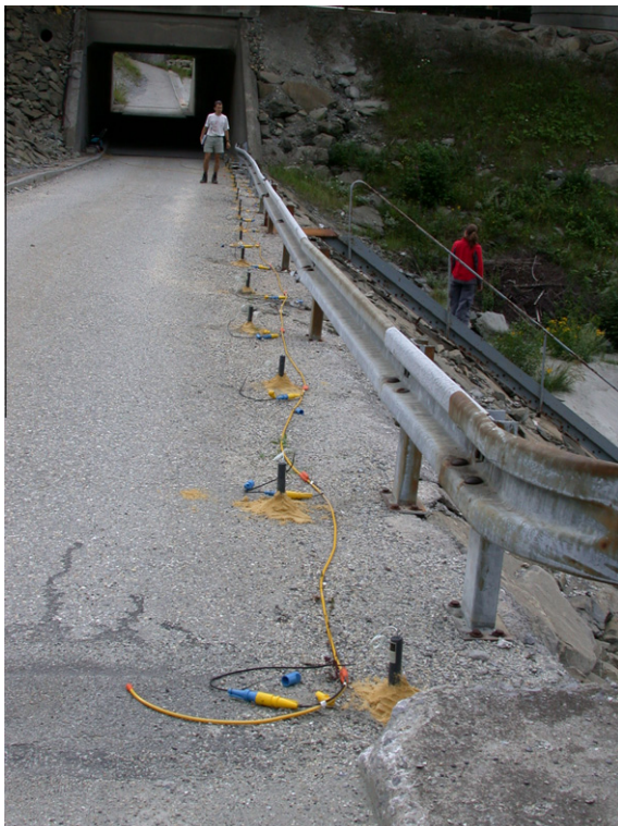
Fig. 8. Self-potential setting. The equipment consists of 2 cables of 16 non-polarizable Petiau electrodes connected to the acquisition system. The self-potential signals are recorded over time with a frequency f equal 200 Hz (signal averaged every second). The electrode spacing is equal to 2 m. In order to improve the electrical contact between the electrodes and the ground, water from the basins was used to decrease the contact resistance.
